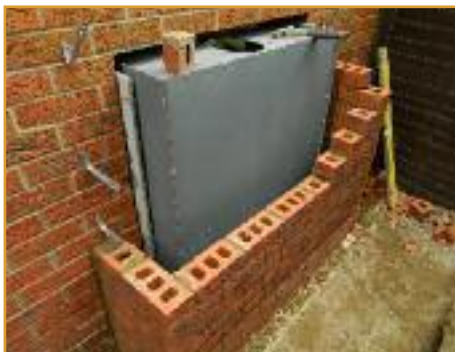
The brickwork is being built around the stove box ready for the insulation mix
