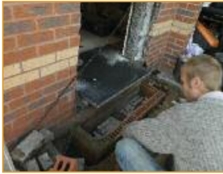
Building from the new foundation up to hearth level.
