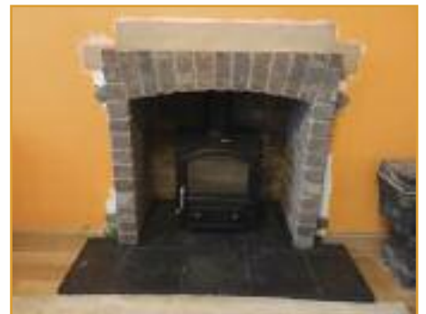
A brick arched fascia has been chosen by the customer ready for the surround.
