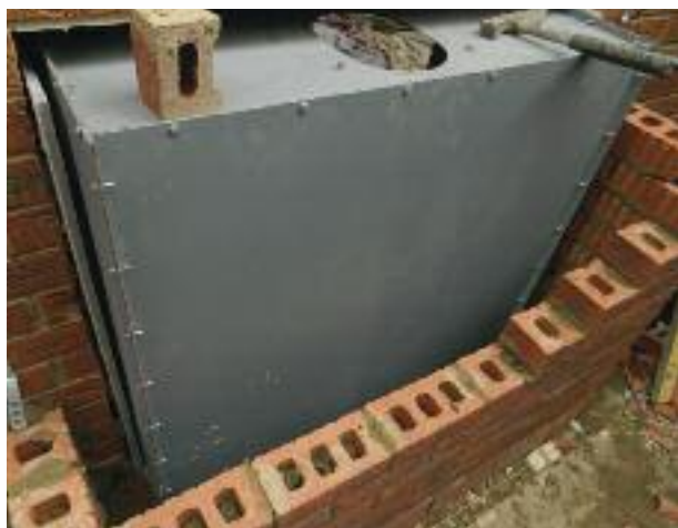
The Eco-Space Saver being installed
