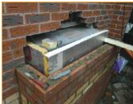
Insulation is being placed in position before the flue is transferred from the stove to twinwall and a new exterior lintel supports the brickwork and the roof angle is formed.
