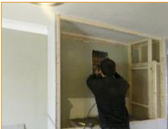
Chopping out for the new flue outlet for the gas stove.
