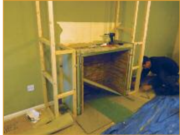
The stove box is placed on the hearth and the false chimney breast is fitted ready for the finish, in this case the customer wanted a plasterboard and skim finish ready to paint.
