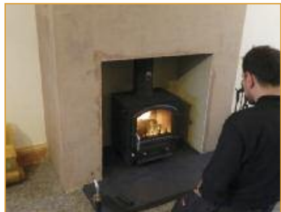
Commissioning the stove, explaining to the customer the controls
