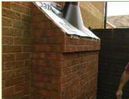
The flue pipe has been transferred from the stove to twinwall and is ready for the roof tiles/flushing.
