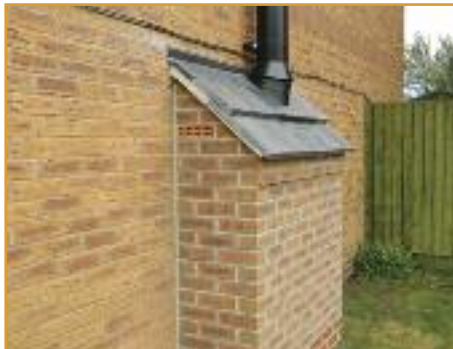
Brickwork and roof tiled ready to take the twinwall up.
