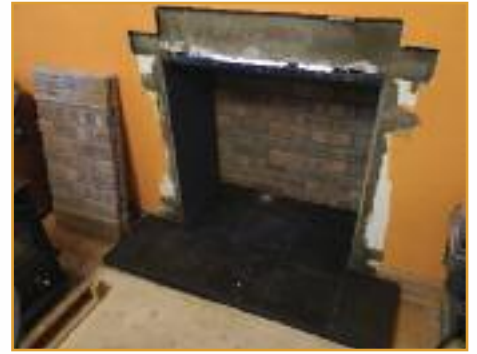
The stove box is fitted and the interior is glued in position and a new lintel has been inserted and rendered.
