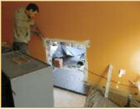
The existing fireplace has been taken out, the foundation has been inspected and filled and the new hearth is in place. Final chopping out ready to insert the SB1 stove box.
