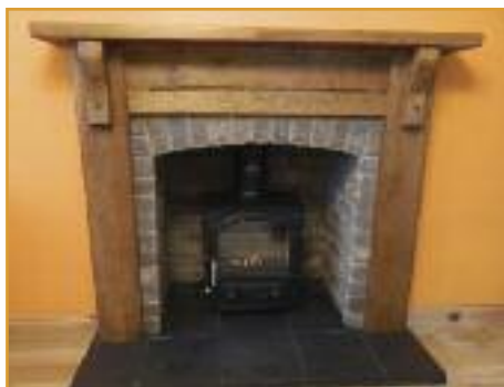
The rustic corbel fire surround in golden oak with the required rebate for the fascia is fixed to the wall to complete the inside fireplace.
