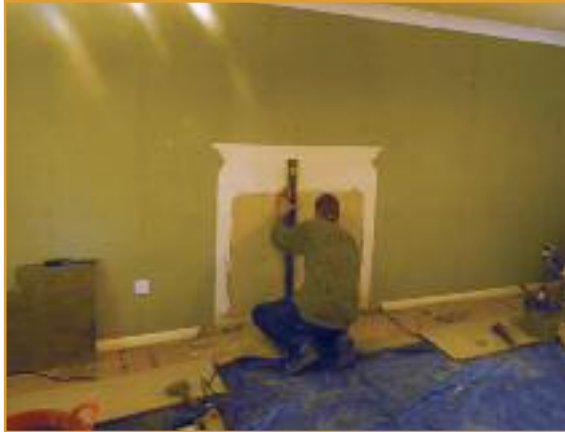
Lining the centre of the new chimney breast
