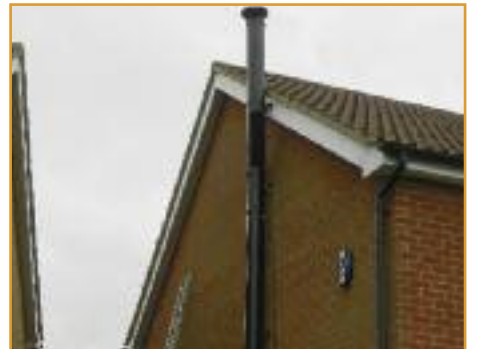
The twinwall has been fitted and completes the work.
