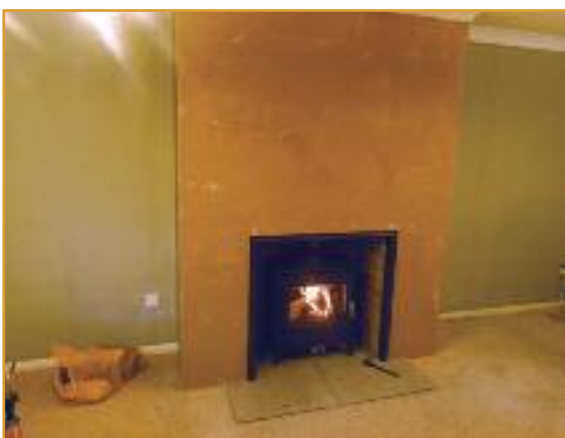
Skimmed and ready for drying to paint
